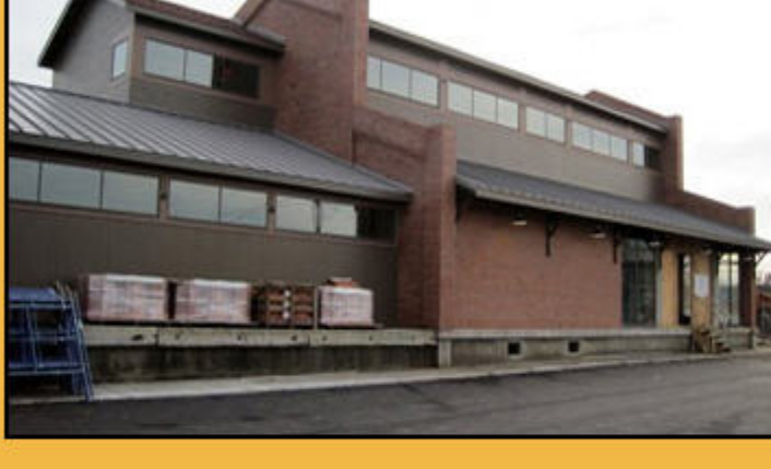
New Muddy Waters Addition, looking west, towards Ground Zero Blues Club
